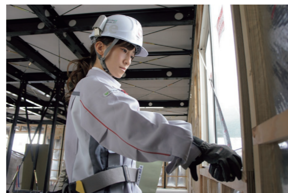
Woman employee supervising construction work at a building site
